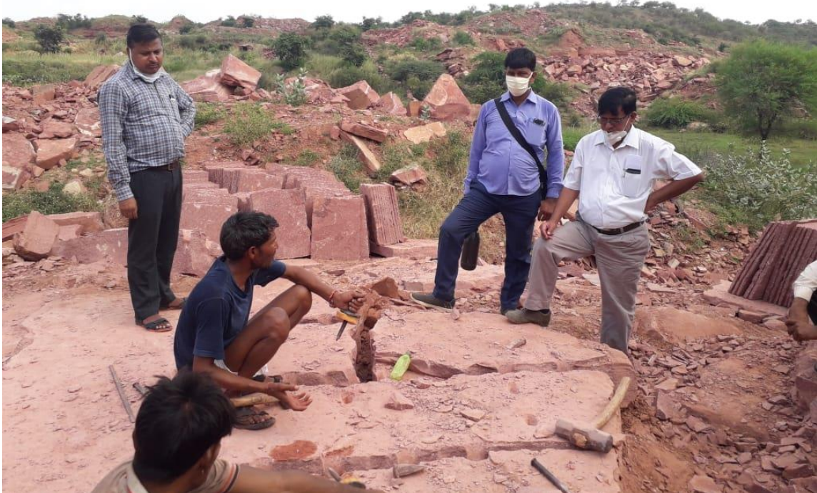
Fig 3 Workers mining stone slab and cut stone slabs in background
